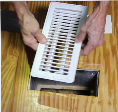
To do: Seal leaky air ducts
