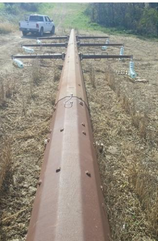
One of the transmission structures set in place for the 345 kV line coming from the Hampton substation.
