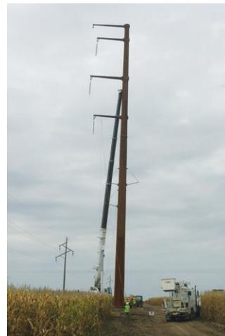
A transmission structure ready to be placed for the 161 kV line from the Chester substation.
