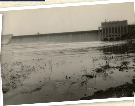
The Lake Zumbro Hydroelectric Dam was designed by Hugh L. Cooper with construction beginning in 1917. It was completed and operational in November of 1919. The facility consists of a powerhouse and a 440-foot spillway across the Zumbro River. Today, the dam can produce a maximum of 2.8 megawatts per hour.
