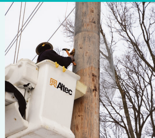
Lineworkers installing wire mesh to the transmission poles behind Mayo Field to prevent woodpecker damage.
