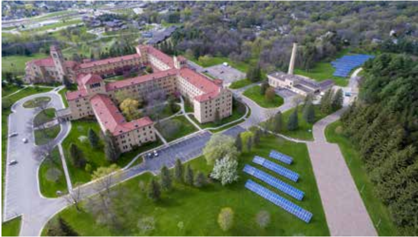
Assisi Heights, 150 kW Solar Rochester, MN
