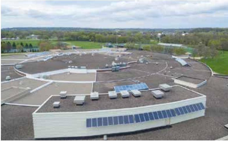
Mayo High School, 5.8 kW Solar Rochester, MN
