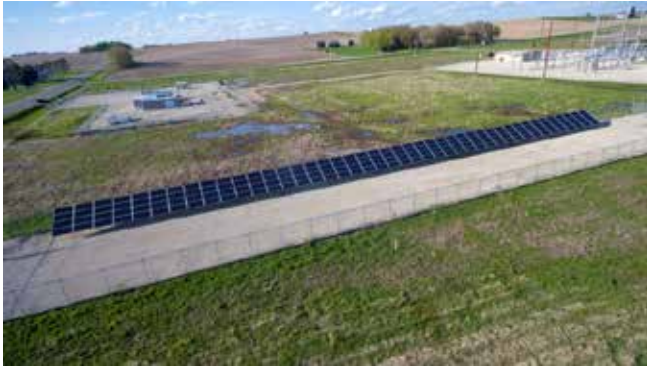
Rochester Public Utilities, 60 kW Solar Westside Energy Station Rochester, MN
