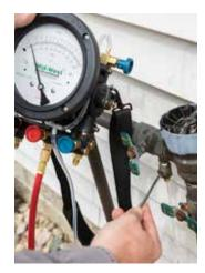
Backflow is the flow of water or other liquids, mixtures or substances, under positive or reduced pressure, into the distribution pipes of a potable water supply from any source other than its intended source. The MN Plumbing Code requires that all backflow preventer assemblies, at the meter and elsewhere within your business or home, must be tested annually by a certified tester.
