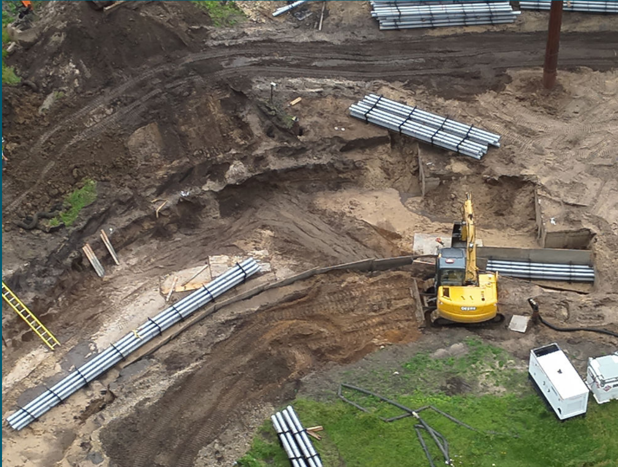
Duct Bank Under Construction
