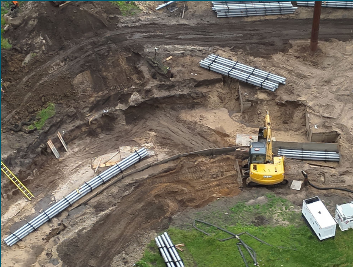
Duct Bank Under Construction
