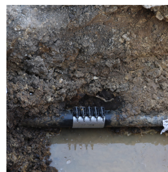
A sleeve is used to repair certain types of water main breaks.
