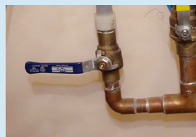
1. An angle valve before the water meter
