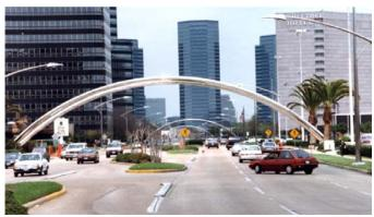
The project called for six pairs of massive arches, which were made of 316 stainless steel. Each unit has a span of 165 feet.
